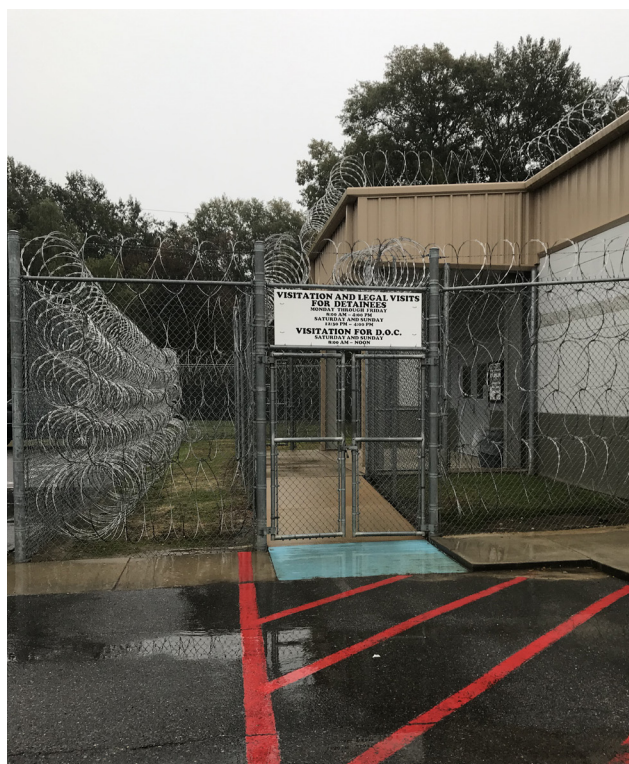
Richwood Correctional Center, Visitor's Entrance
